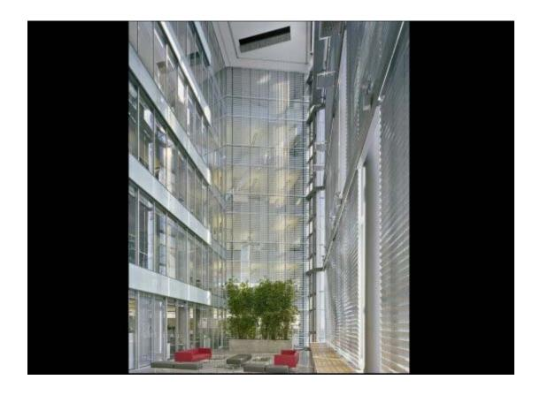
Twenty-one stories tall and with 695,000 square feet of space, the corporate headquarters of the Manitoba electricity and natural gas utility is one of the greenest, most-energy efficient buildings in the world. The building is sited to take maximal advantage of prevailing winds and solar energy. Green roofs use plants to reduce stormwater runoff; waterfalls humidify the interior and a solar chimney provides fresh air.
